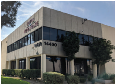
LOTUS & WINDOWARE - CHINO, CA Corporate Office | 45,000 Square Foot Warehouse
